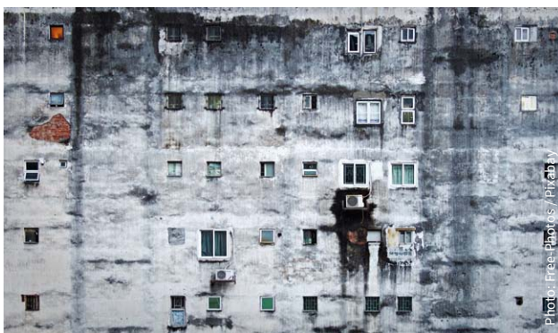
A poorly constructed house for the financially poorer people.
