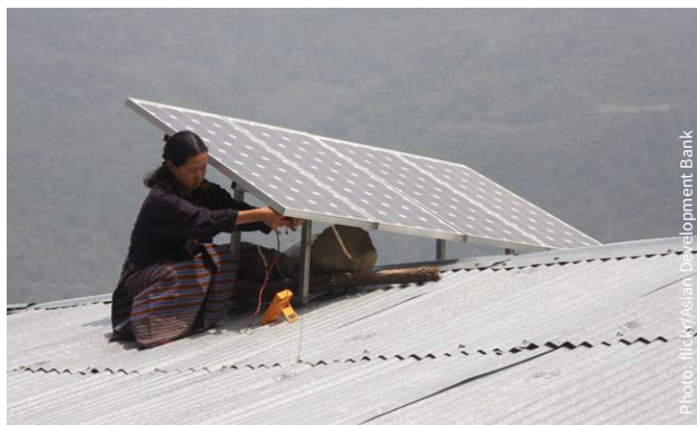
Sustainability right from the start: The installation of solar panels in Bhutan
