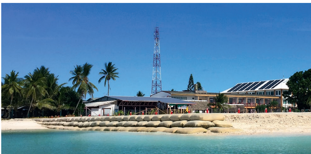
Measures to adapt to climate-related sea level rise by building artificial sea walls in Tuvalu, South Pacific
