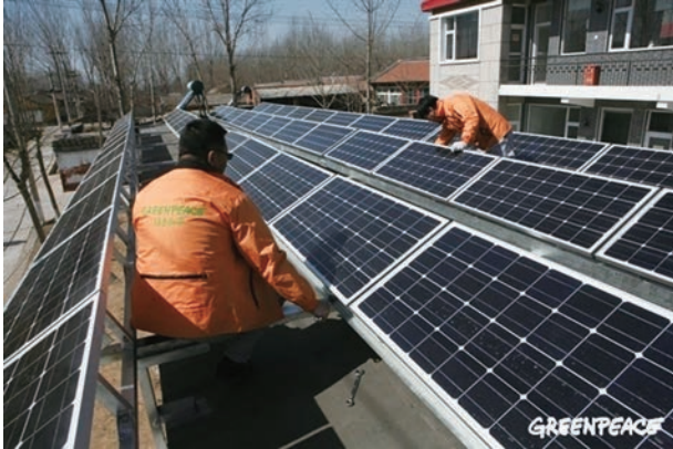
Greenpeace's solar installation
