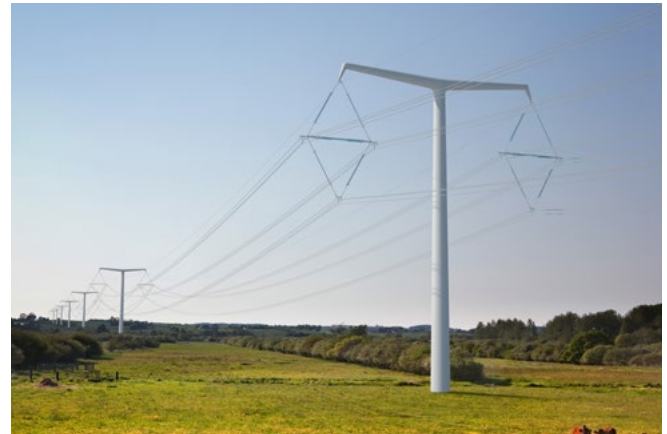
T-pylon / Photo: National Grid
